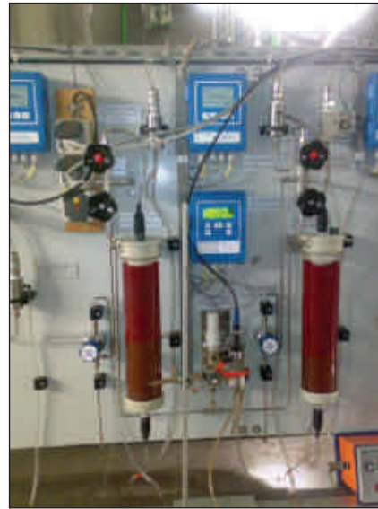
Figure 9: Random arrangement of flow cells and transmitters.
