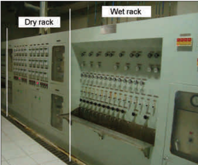
Figure 2: Front view of a sampling system with wet and dry rack sections.
